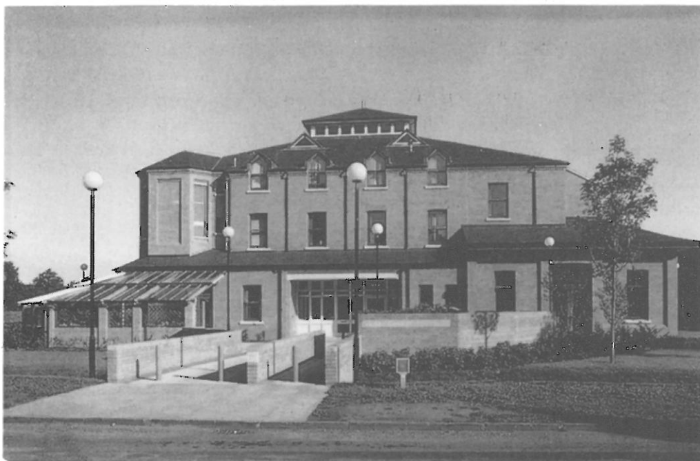
The Newton Institute building designed by Annand & Mustoe
