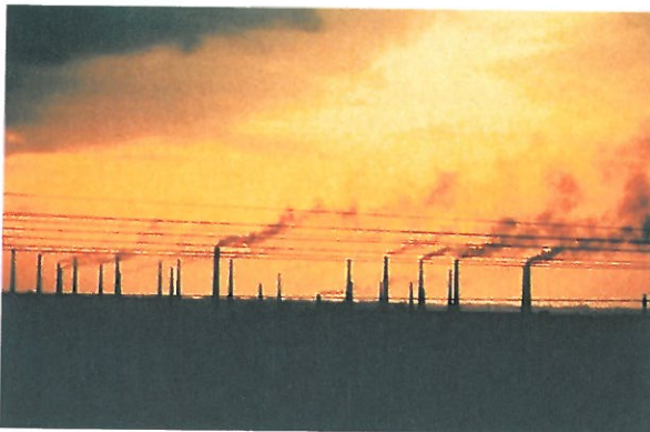
Brickworks at dusk (Woburn, Bedfordshire). By day, smoke is carried freely up and down by the motion of the air when there is any thermal convection from the ground. At sunset, when the cooling of the ground has stabilised the lower layers of air, they are much less turbulent. The heat of the gases carries the plumes of smoke upwards in the neutrally stratified air at higher levels and no odour reaches the ground.
