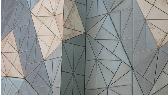
Figure 3: Aperiodic pinwheel pattern on a building in Federation Square, Melbourne. Tiled on the plane, the triangles appear in an infinite number of rotations. Photo by M Subritzky
